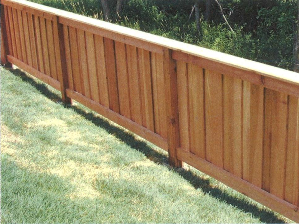
Figure 3: Board-on-Board (wood)
