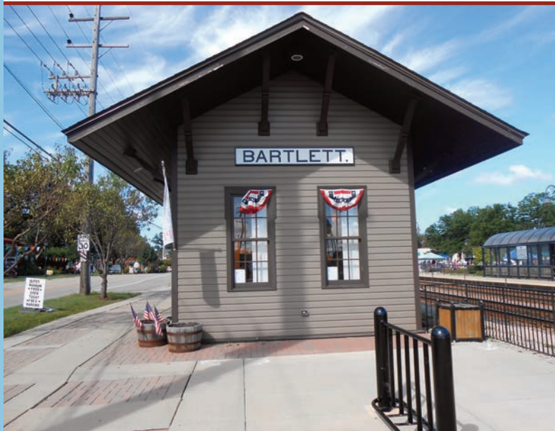
The Bartlett Depot Museum, built in 1873, is located at 100 W. Railroad Avenue.
