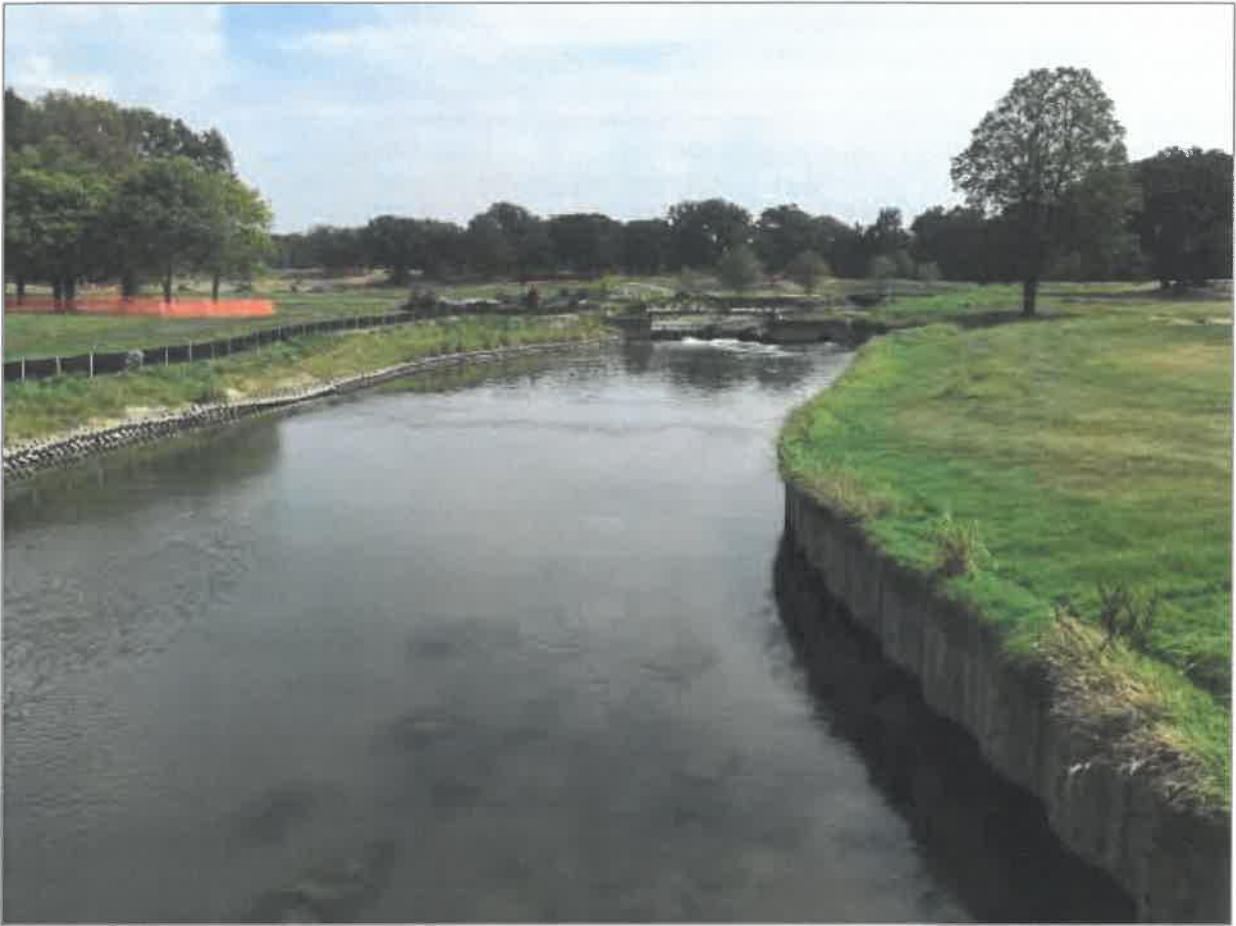
Plate 2. Pre existing conditions downstream of the principle dam at RM 22.7 looking north. The ubiquitous A-Jacks (viewer's left) and sheet piling (viewer's right) are clearly visible.
