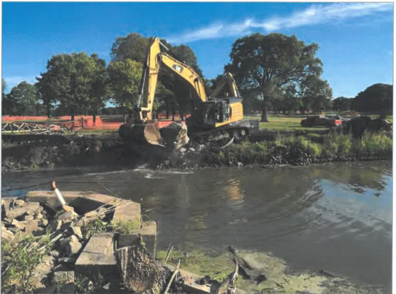
Plate 3. Deconstruction of the dam at RM 22.7 (image FPDDC).
