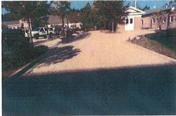
① Northeast entrance looking west at parking lot pavement.
