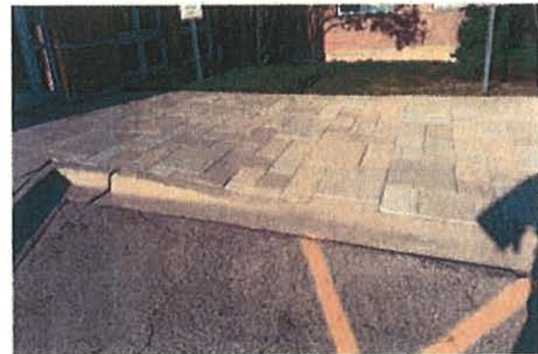
⑥ Looking west at brick pavers at ADA entrance.
