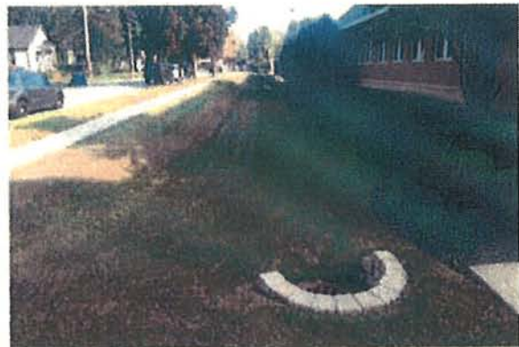
② Looking north at the detention basin.
