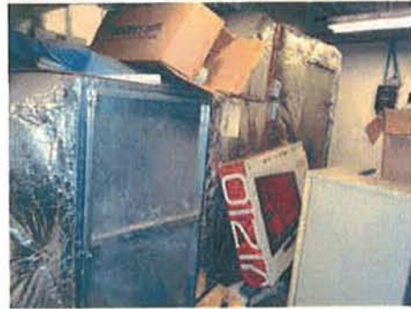
HEPA filtered exhaust for firing range
