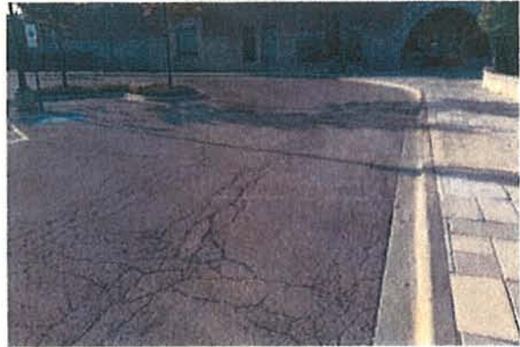
⑧ Looking south at parking lot pavement
