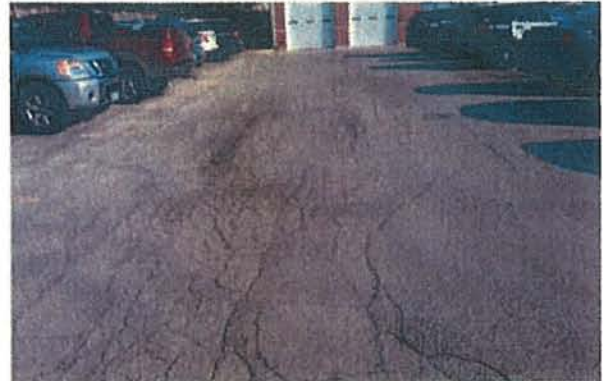
8 Looking north at the pavement of the police lot
