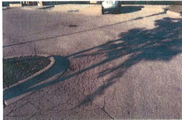
③ Looking northwest at parking lot pavement
