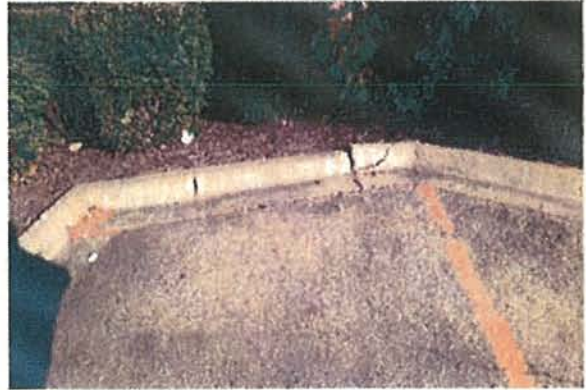
⑭ Looking northwest at existing curb in the main parking lot
