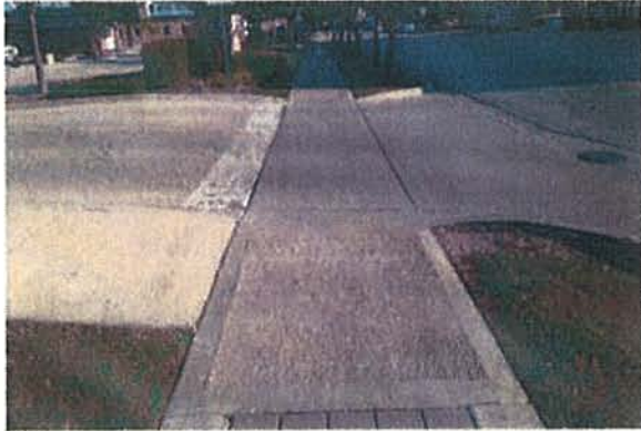
⑬ Looking north at the existing sidewalk and ADA crossing.
