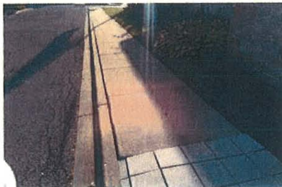
⑪ Looking east at the sidewalk along the back of curb
