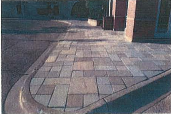
⑦ Looking south at brick pavers in island nose.
