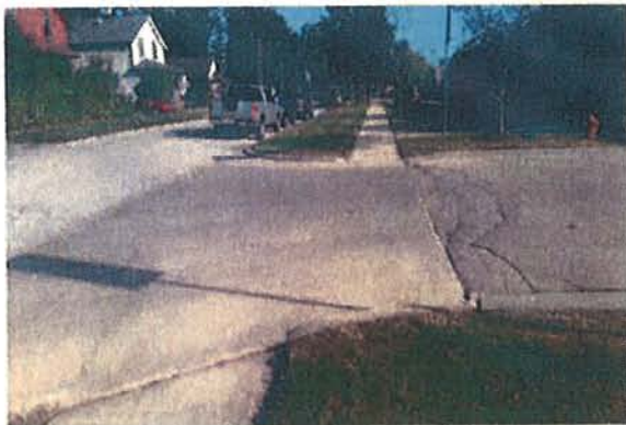
① Looking north at the west entrance to the employee lot.
