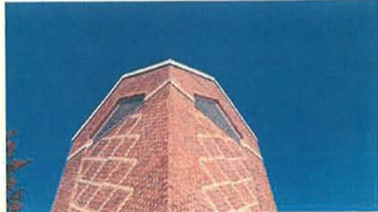
Louvers for RTU inside Tower
