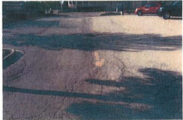
② Looking south at parking lot pavement.
