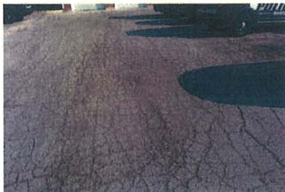
9 Looking north at the pavement of the police lot
