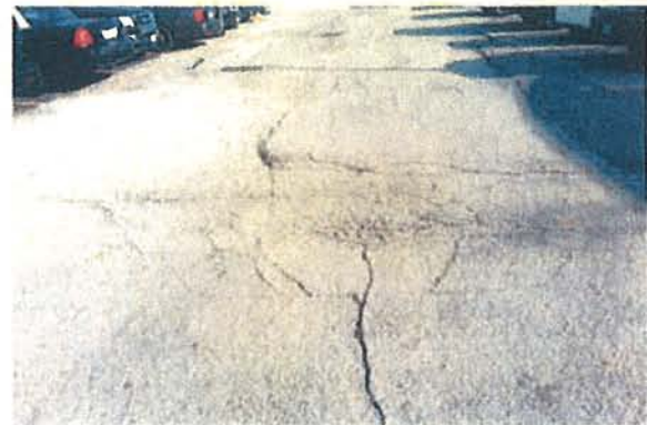
10 Looking north at the pavement of the police lot
