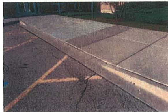
⑤ Looking southwest at ADA entrance
