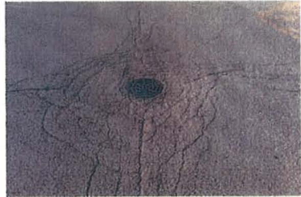
④ Pavement around drainage structure in center aisle.
