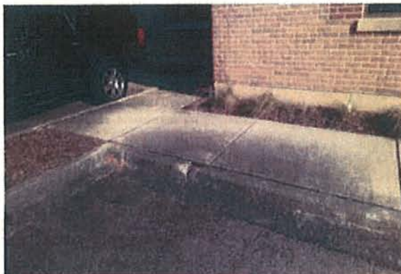
⑰ Looking northwest at the curb/sidewalk in the employee lot.
