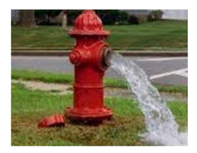
It's time for Bartlett Public Works to flush all fire hydrants. This process removes iron deposits from the water mains and ensures that hydrants are working correctly.
