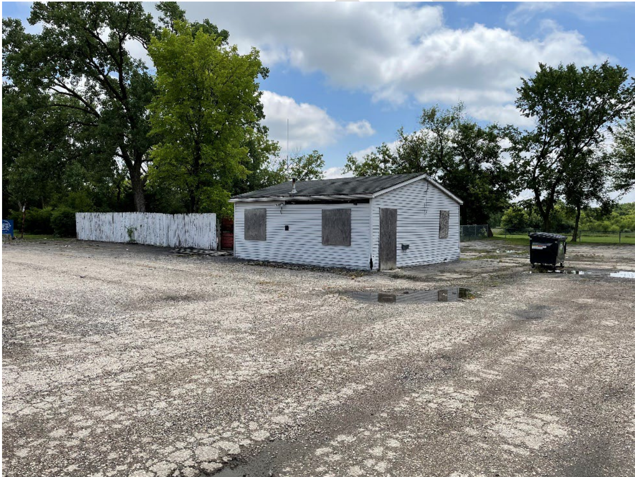
ABOVE: Examples of Deterioration observed during field survey. Source: Teska Associates, Inc.
