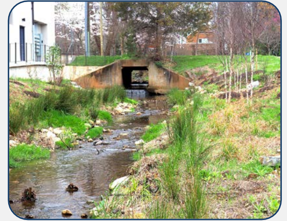
Floodplain bench and rock toe
