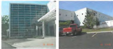
High quality exterior facade materials include metal siding, clerestory glazing and brick masonry. High quality landscape plantings provide for usable outdoor space by employees and visitors.
