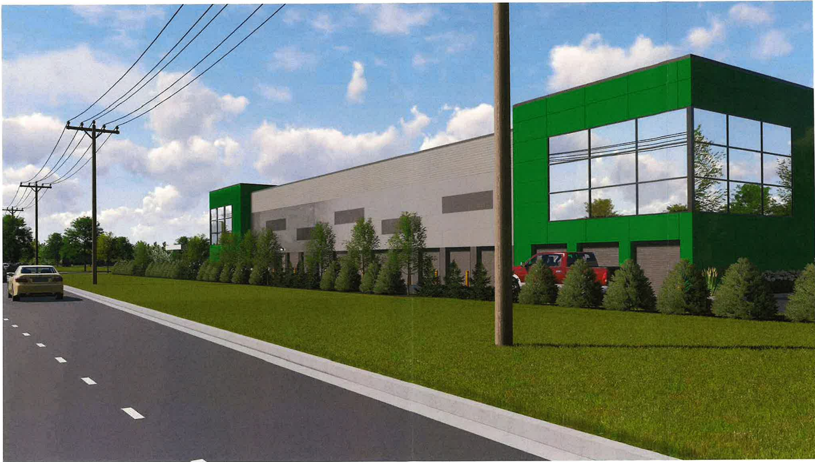
VIEW FROM NORTHEBOUND ROUTE 25
