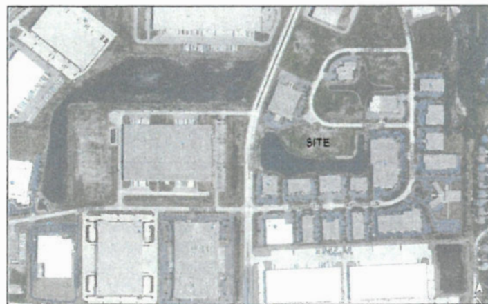
BUILDING AERIAL VIEW NORTH NO SCALE
