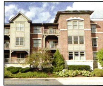
Adjacent 3 ½ - 4 Story Multi- Family Building
