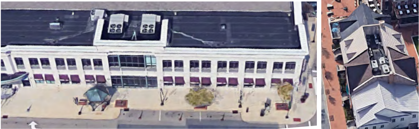
Figure 22. Rooftop Utilities Screened from the Public Way by a Parapet on left and Pitched Cap on right
