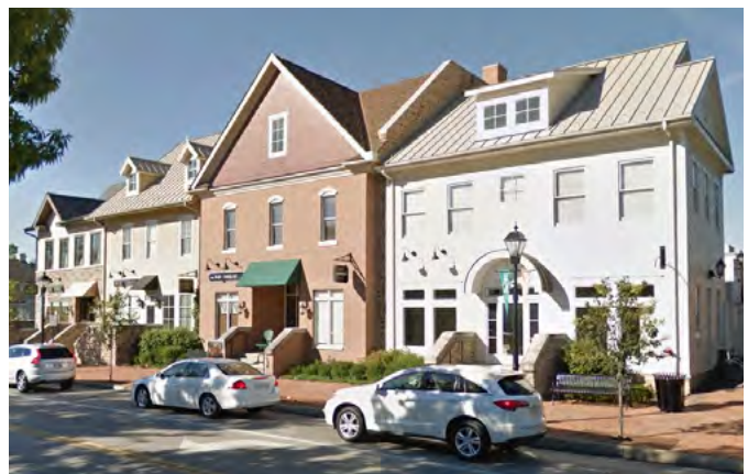
Figure 19. Example of Building Facade Variety and Articulation of Stories
