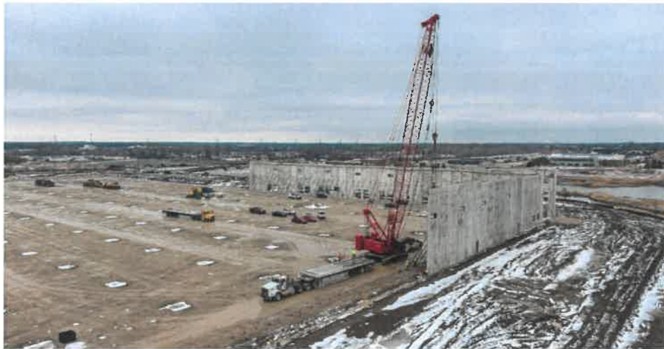
Conor Globe Commercial's new facility underway
