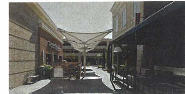
Figure 32. Examples of Pedestrianways between Buildings
