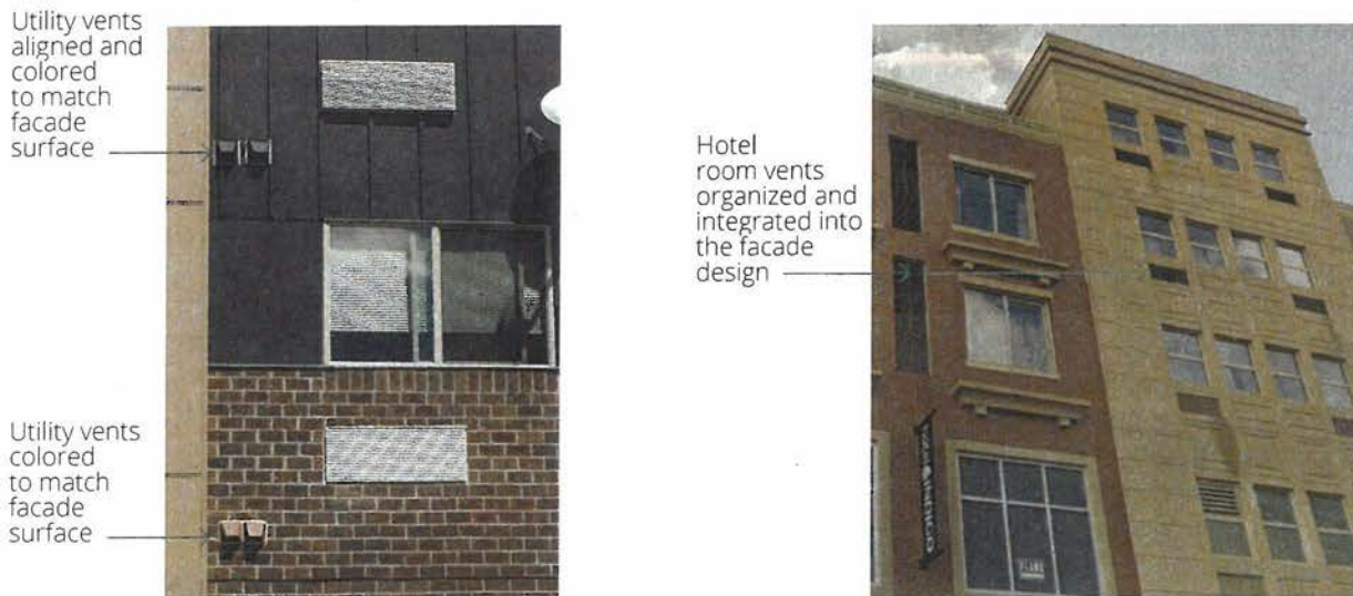
Figure 23. Utility Appurtenances located on Facades
