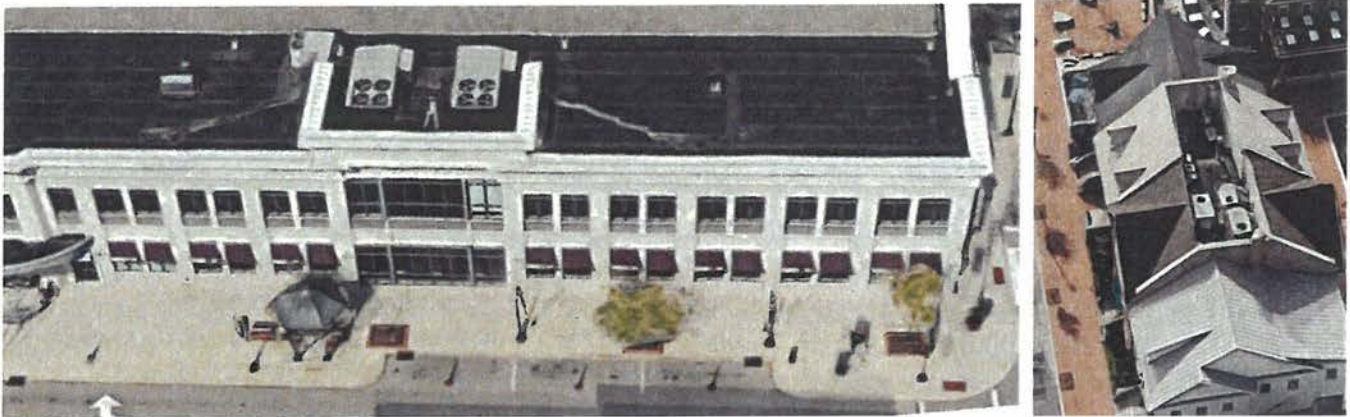
Figure 22. Rooftop Utilities Screened from the Public Way by a Parapet on left and Pitched Cap on right
