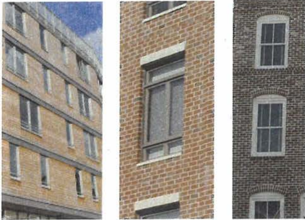
Figure 14. Vertically Oriented Windows with Expressed Lintels
