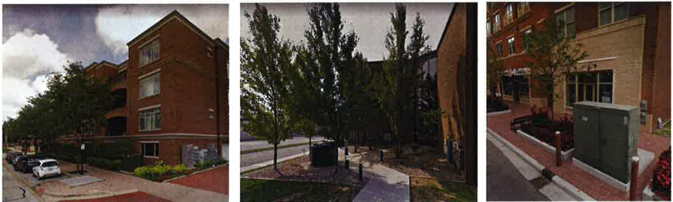
Figure 24. Examples of Poorly Located Utility Appurtenances without Screening on Primary Streets: NOT PERMITTED
