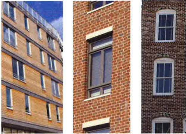
Figure 14. Vertically Oriented Windows with Expressed Lintels
