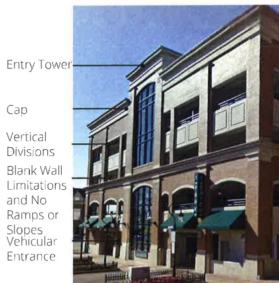
Figure 25. Example Parking Structure fronting a street
