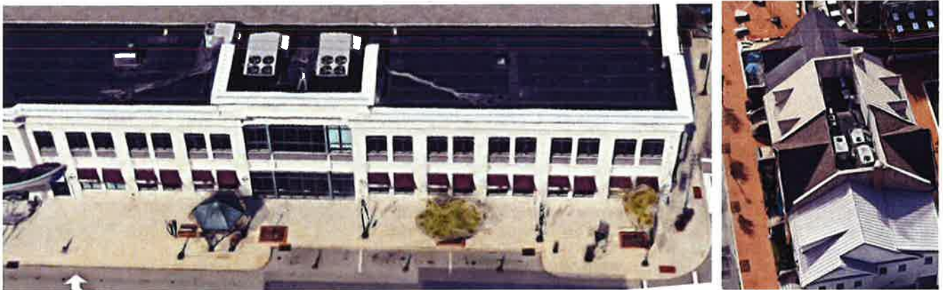
Figure 22. Rooftop Utilities Screened from the Public Way by a Parapet on left and Pitched Cap on right
