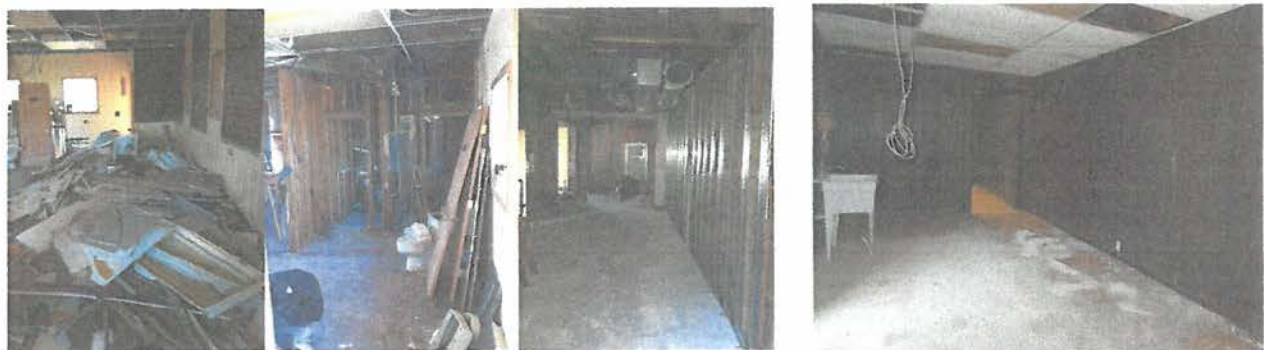
Dining Room, bathroom, kitchen and office prior to improvements
