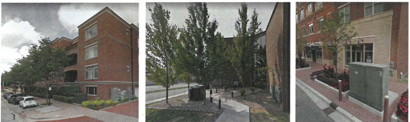
Figure 24. Examples of Poorly Located Utility Appurtenances without Screening on Primary Streets: NOT PERMITTED
