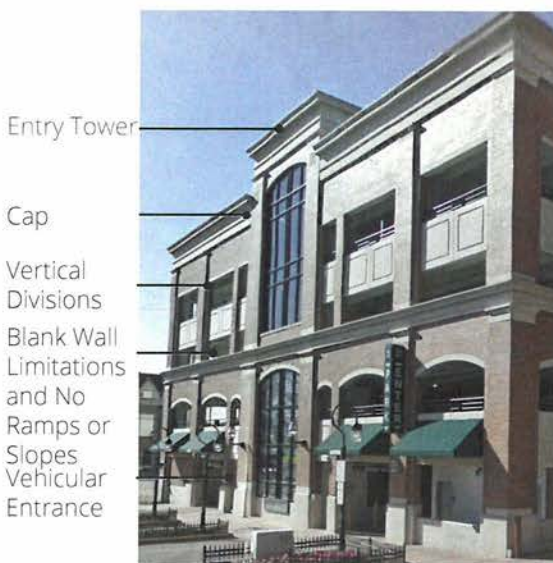
Figure 25. Example Parking Structure fronting a street
