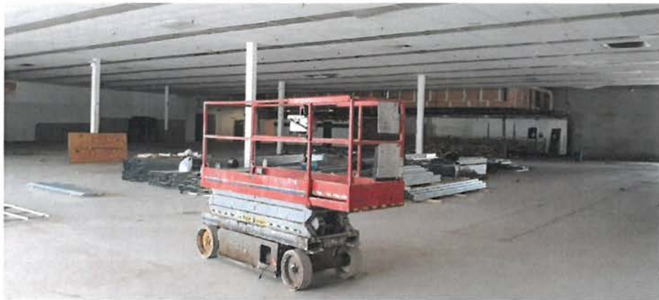
Interior of former grocery space
