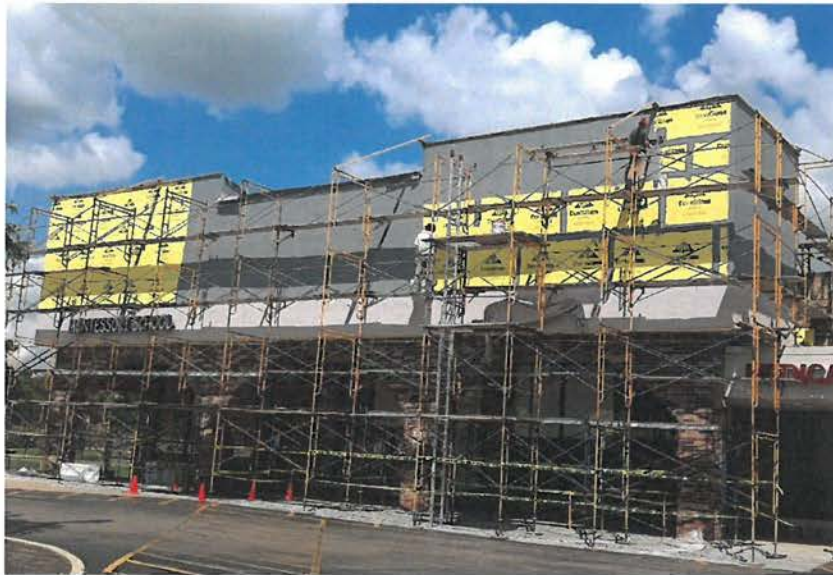
Facade renovations underway
