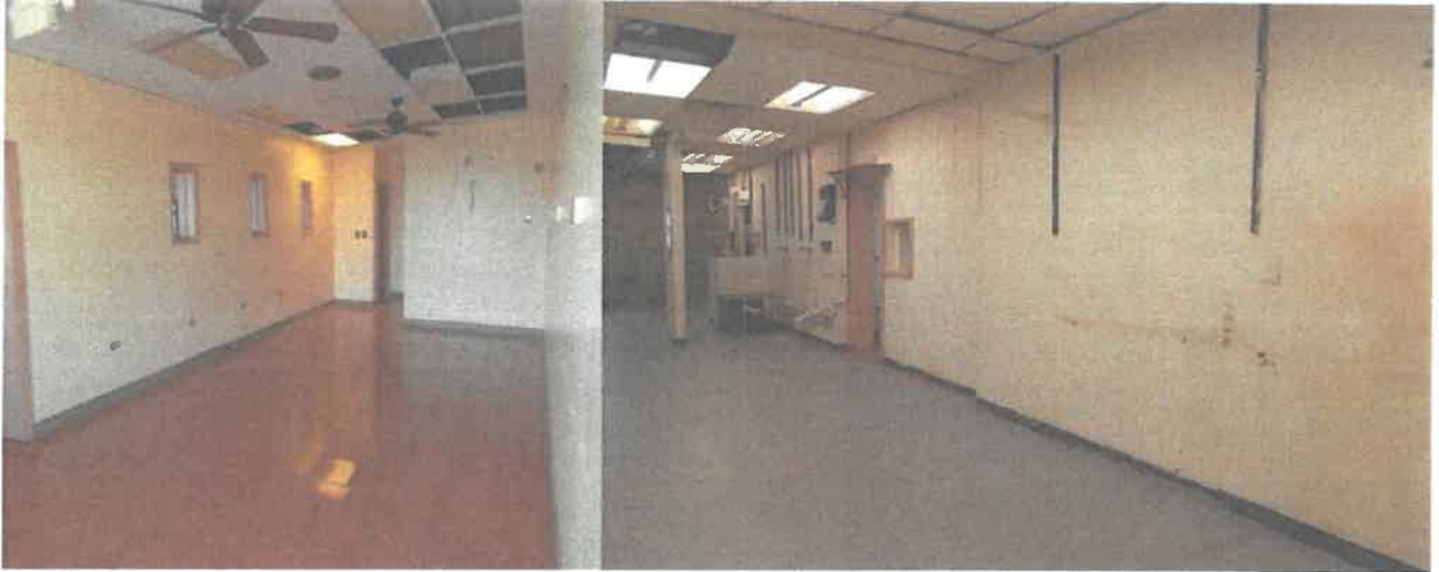
Bar and Kitchen Space Prior to Remodel
