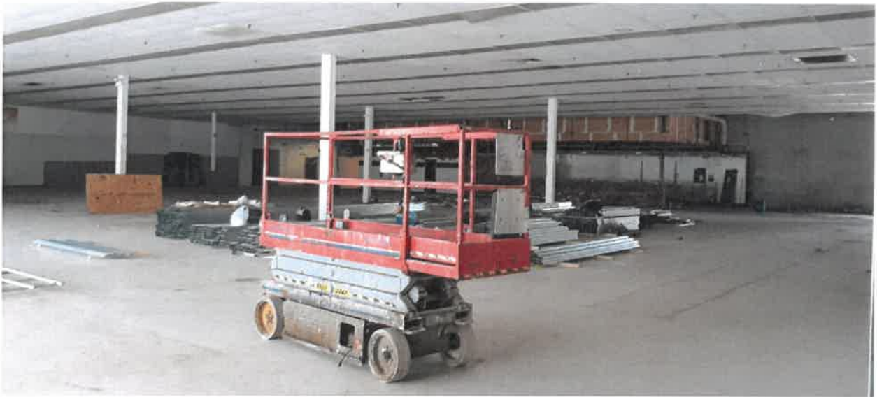
Interior of former grocery space
