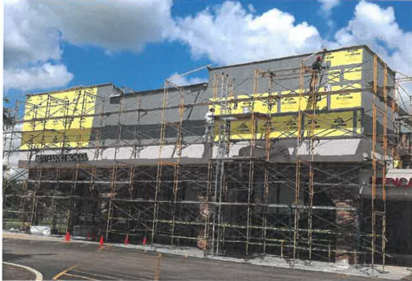
Facade renovations underway
